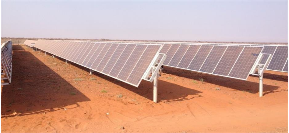
Figure 5-8: A single axis tracking system
