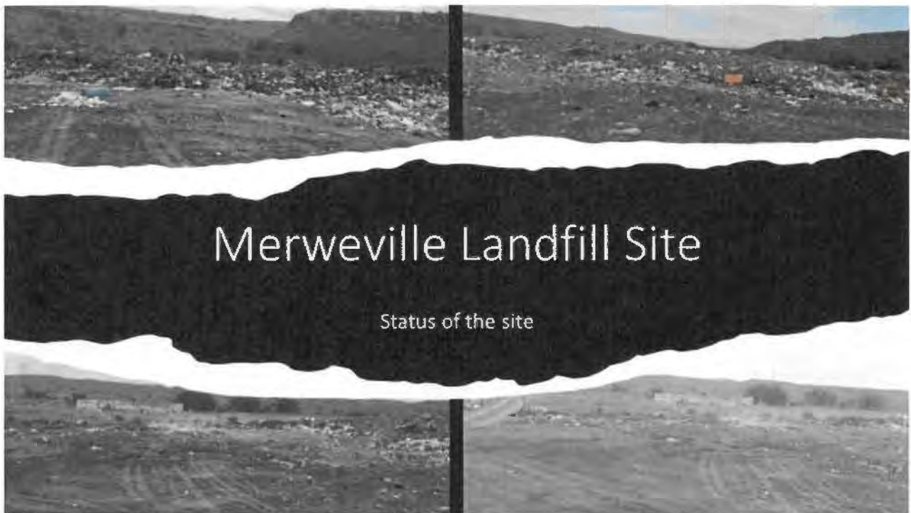
Figure 4-17: Status of Merweville Waste Disposal Facility
