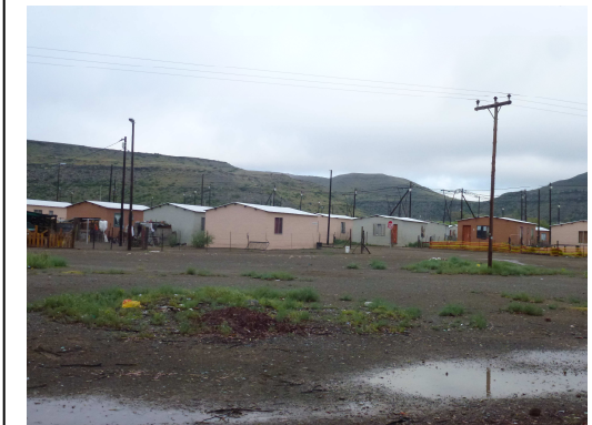
Recently constructed BNG housing
