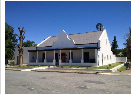
Former building on corner Parsonage and Sir George Grey Streets previously in poor condition when used as a shop (Google Street view 2010). Now restored and used for its original purpose
