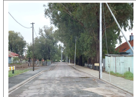
Replace existing blue gums with indigenous trees on phased basis so as to retain visual quality
