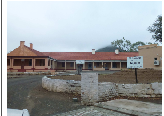
Example of numerous well built but little used institutional buildings on site requiring maintenance
